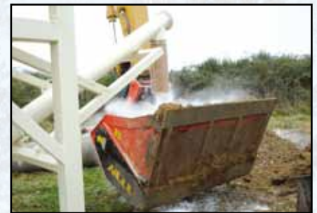
Stabilising soil with lime
