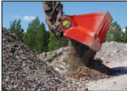
Crushing bricks / black top asphalt
