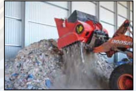
Crushing demolition waste
